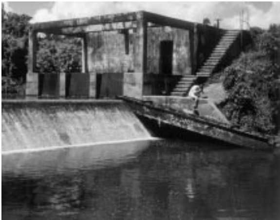
PLATE 1. The Espiritu Santo dam and water intake, July 1995. Note the defunct fish ladder below, and the triple-barred intake above the dam sill on the right. Photograph by Catherine Pringle.
